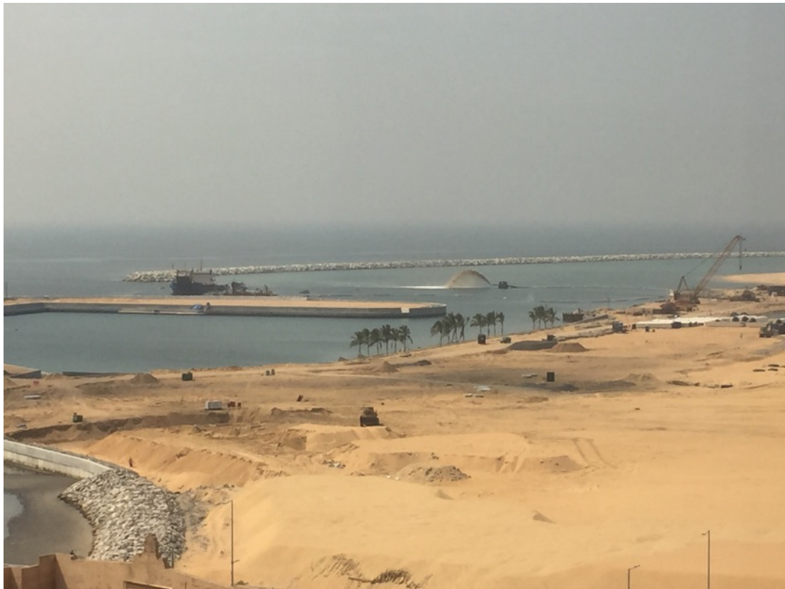
Land filling operations – the expected ground of Colombo Port City. December 2019
